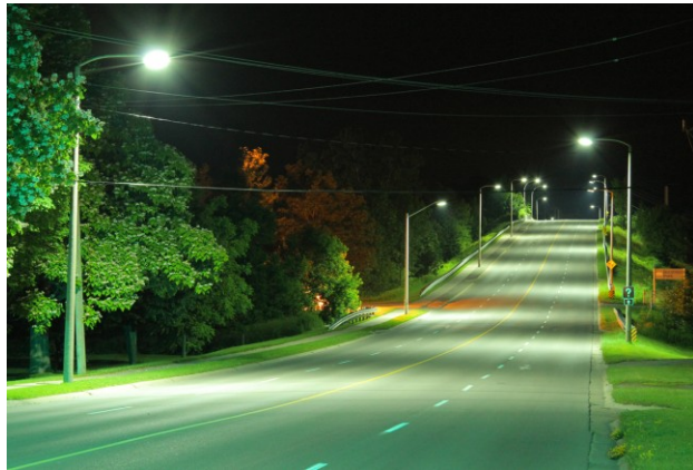
Figure 3.48 - This tiger-stripe lighting pattern on the roadway due to the FCO induction street-lighting in Brockville, Ontario, would have been unthinkable more than a decade ago. Such are the powers of the lighting industry that anything can be marketed in support of a supposed cost-cutting measure.
