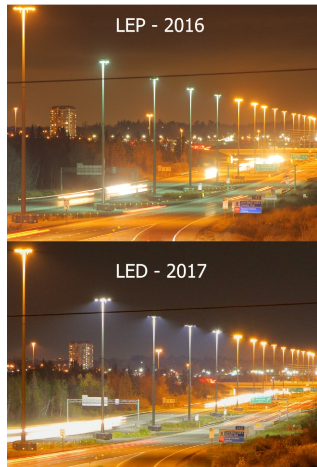
Figure 2.45 - On a stretch of Highway #417, in Kanata, west of Ottawa, Ontario, there were 4 masts with LEP lighting units that were being evaluated. The blue-green light they emitted (top image) was in stark contrast with the orange light from the HPS masts. By the end of 2017, these were replaced with new LED luminaires (bottom image).
