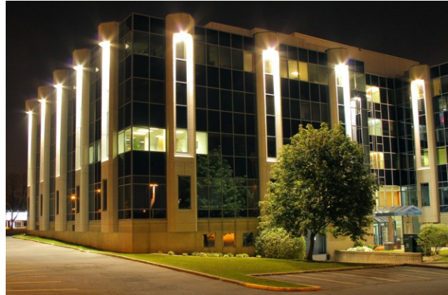
Figure 3.72 - Excellent down-lighting with metal-halide lamps judiciously conceived when this building was constructed, the lamps supplying light for pedestrians and for the parking lot.
