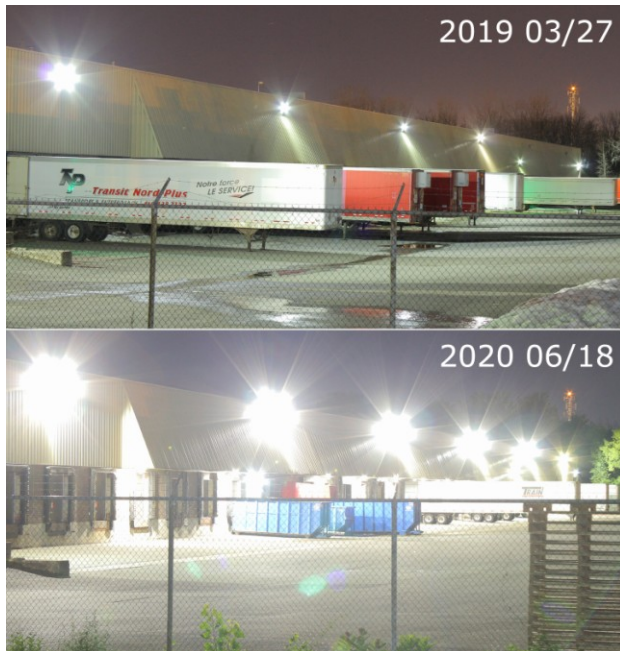
Figure 7.10 - With a pair of LED system units replacing failed units in the distance (at right), light levels soared when all the metal-halide flood lights for this industry lot were replaced. According to the exposure settings, a fourfold increase in the light level was estimated: to match the two histograms of the images the ISO had to be changed from 1250 to 320 ISO.
