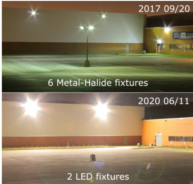
Figure 7.9 - Many older metal-halide perimeter lights are now being replaced with new and powerful LED systems. The same lot was photographed nearly three years apart with the same camera settings. The newly installed LED wall-packs are more polluting than previously with just two luminaires.
