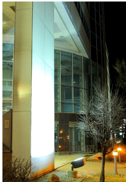
Figure 3.71 - The 1000 watt MH floodlight shown in Figure 3.70, one of six such fixtures, is illuminating a column of a building. This was photographed in March of 2019 and the fixture appears to have one third of its light sky-bound.
