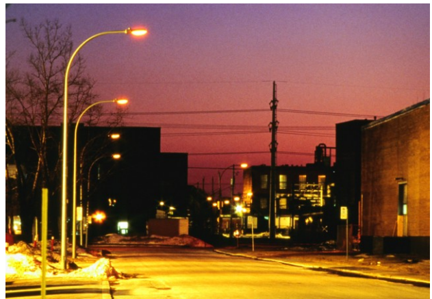
Figure 3.51 - Low pressure sodium (LPS) street-lighting using semi-cutoff type heads with 55 watt lamps. These have nearly the equivalent mean lumen output as 100 watt HPS lamps.
