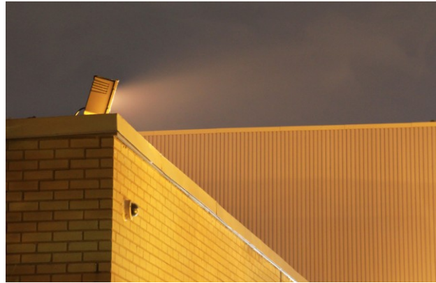
Figure 4.34 - Typical lot lighting fixtures have about 25% direct up-light. This single 400 watt flood-light pollutes like thirty-two 100 watt HPS older cobra-heads for urban settings.
