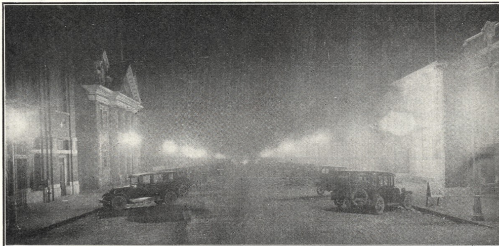
NIGHT SCENE IN SOUTH BEND AFTER SINGLE-LIGHT STANDARDS WERE INSTALLED
