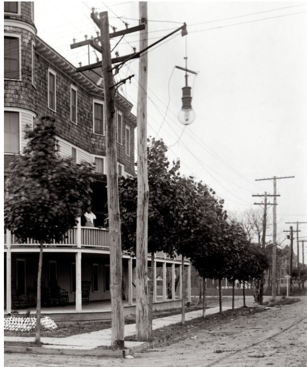
Figure 3.4 - For easy maintenance and relamping, the earliest series incandescent lamps were also installed on masts with winching systems. Rope tied near the base of the post was released to lower the lamp. Severn Hall hotel in Wildwood, New Jersey, circa 1907, part of an 8x10 inch dry plate glass negative, Detroit Publishing Company.
