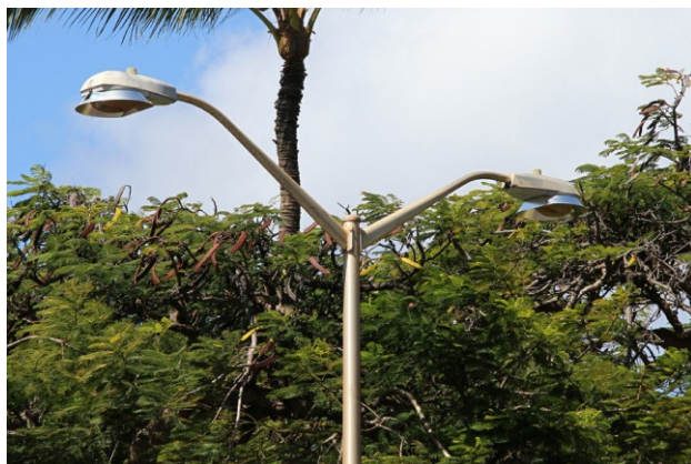
Figure 3.49 - In certain sensitive areas, such as on some Hawaiian islands, old cobra heads were shielded making them into cutoff heads from semi-cutoff and non-cutoff type.
