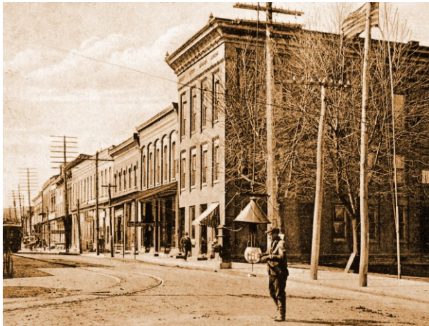
Figure 3.3 - Many arc-lamps were installed on intersections on a mast with a winching mechanism. An arc-lamp is lowered here by a worker for maintenance. The earliest arc-lamps required daily cleaning and rod replacement. From a 1905 postcard, W. A. Reed, Stationer, Milton, Pennsylvania.
