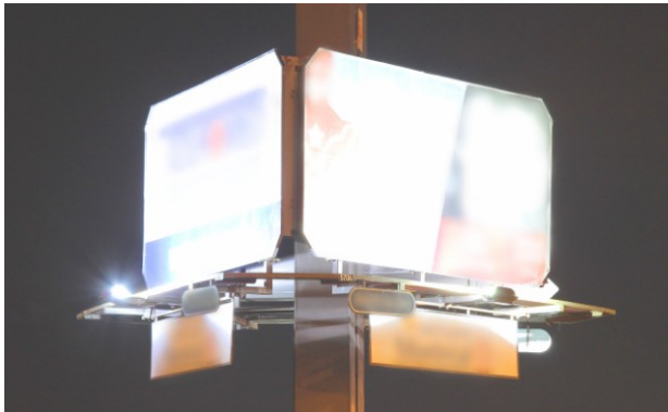
Figure 4.37 - Up-turned billboard lamps shed most of their light directly into the night sky. Therefore, the metal-halide spectral signature from these billboards (or LED for modern billboards) must be apparent in the night sky spectrum.
