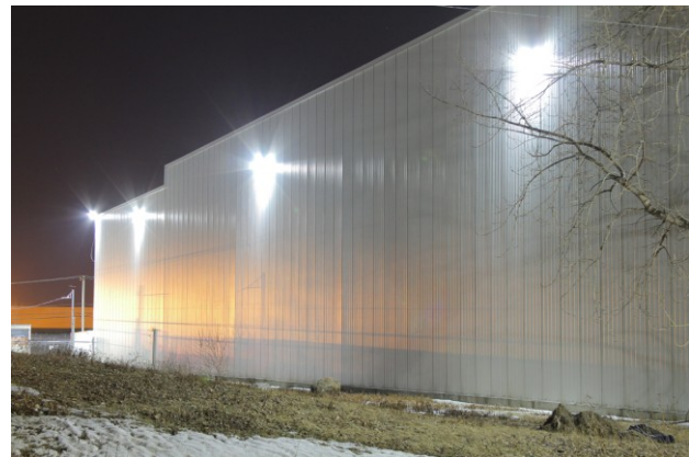
Figure 3.73 - Wall-packs on the rear of a building confounding the viewer as there are no exits or entries, nor a parking lot or landscaping, except perhaps for a single emergency exit.
