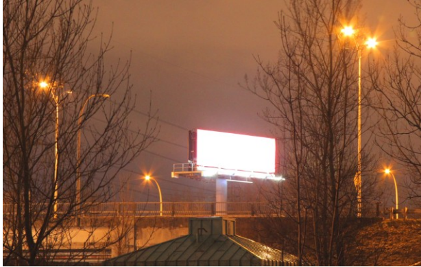
Figure 4.36 - The five 400 watt metal-halide billboard lamps (~67% up-light) that are facing us, pollute like forty-three 250 watt FCO HPS luminaires located on the very same highway (with 10% up-light for an industrial setting and no canopy).
