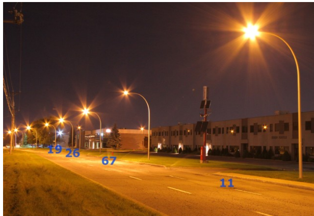
Figure 4.33 - For whatever reason, when a classic cobra-head was replaced with a FCO one, the watts often remained the same. Compared to the former light levels, the new levels below a FCO street-light (second from right in this image) became double or more. The measured lux values are marked below four HPS heads, all of which showed a "25" NEMA tag.
