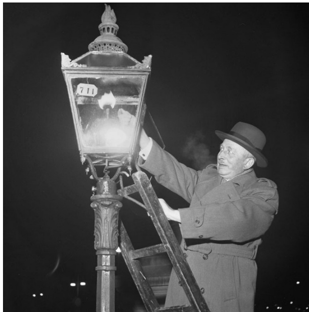
Figure 2.4 - Early gas lanterns had to be ignited manually. A naked-flame gas burner is lighted here by a lamplighter in Sweden, in 1953. By this time, such remaining gaslights were uncommon curiosities. This photograph is in the public domain in its country of origin and many other countries.
