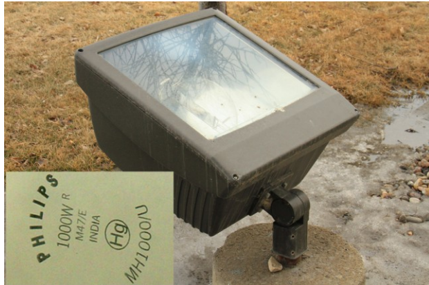
Figure 3.70 - A large one meter squared (3' x 3') fixture with a kilowatt MH lamp is pointing upwards. The insert shows the lamp's etch. This fixture is also shown in Figure 3.71.
